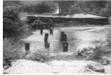
Excavating the stream may lead to infrastructure loss
