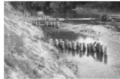
Seek expert advice if installing bank stabilisation structures such as pin groynes
