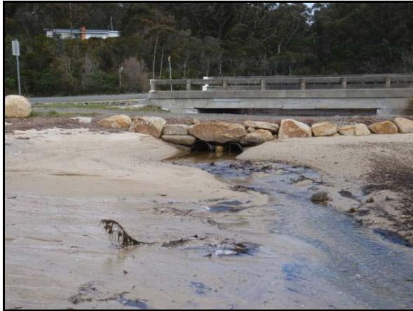
Figure 144.4. Restricted flow through pedestrian walkway.
