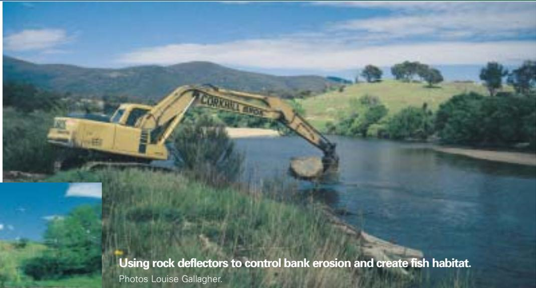
Using rock deflectors to control bank erosion and create fish habitat.
